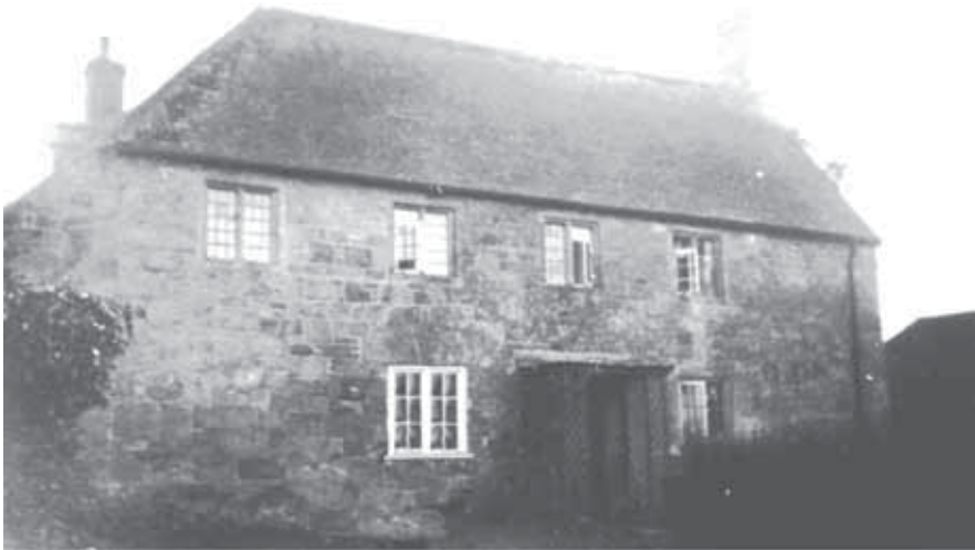
Figure 2: Sweetwell Farm (now demolished)
